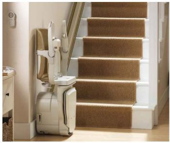
**With its narrow rail** and slim design, this stairlift takes up little room. A remote at each landing allows the chair to be called or sent away.
